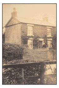
A typical nineteenth century house built in brick with a slate roof. Note the large sliding sash windows and the central front door.
